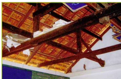
Above: Korn Pissey High School, the library shelf is situated in the rafters.
