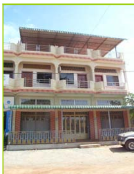
Above: The outside of the café will in time be an alfresco area. The Internet Café occupies the ground floor of HOP.
